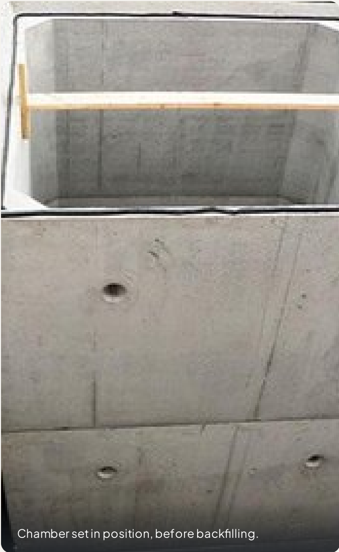
Precast chamber with a connection opening.
